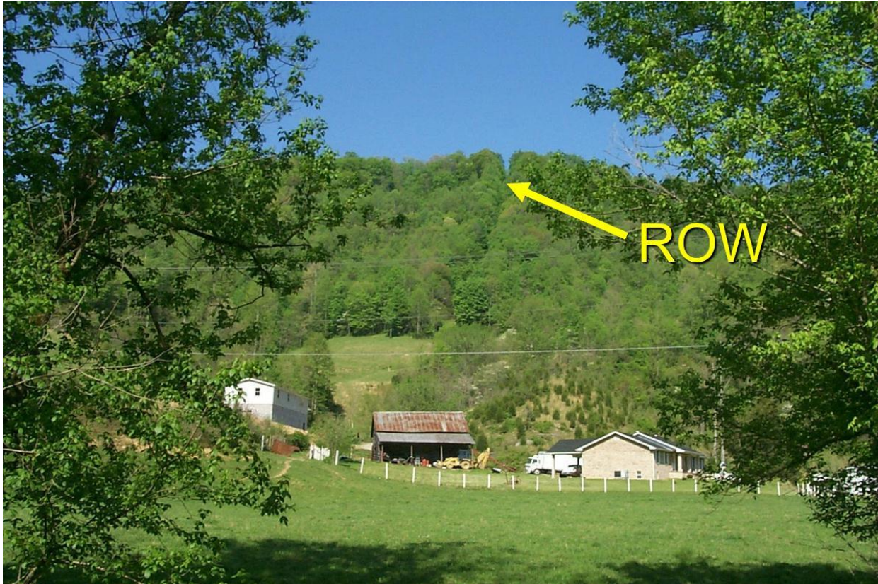
Figure 2. A 40 year-old pipeline ROW has remained visible through vegetation maintenance.
