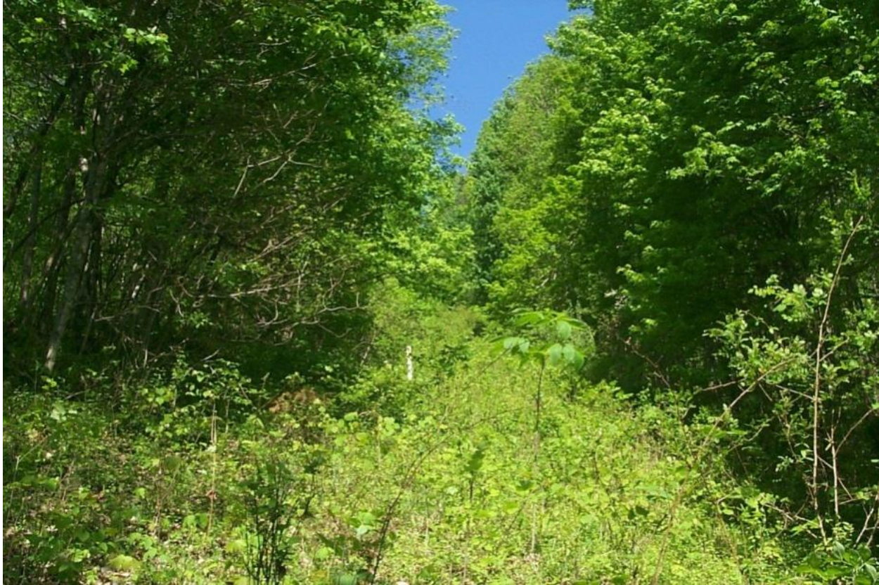
Figure 5. A 50 foot wide pipeline ROW overgrown to a width of 30 feet.
